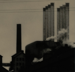
4 Michigan Finest Headquarters Ford Rouge Plant (from Dix Rd. Bridge) Russ Marshall
